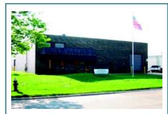
Amphenol Power Solutions in Fraser, MI houses the manufacture of RADSOK® and power cable products.
